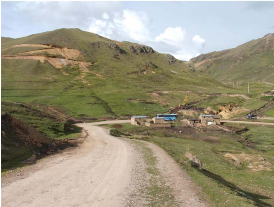
Photo 1. Looking NNE with diamond drill rig drilling by the public access road
